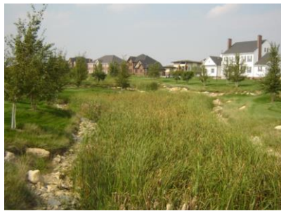
Example of a Drainageway or Surface Drain
