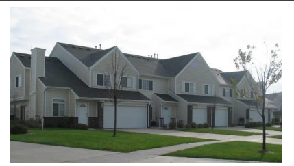
Example of Single-Family Attached
