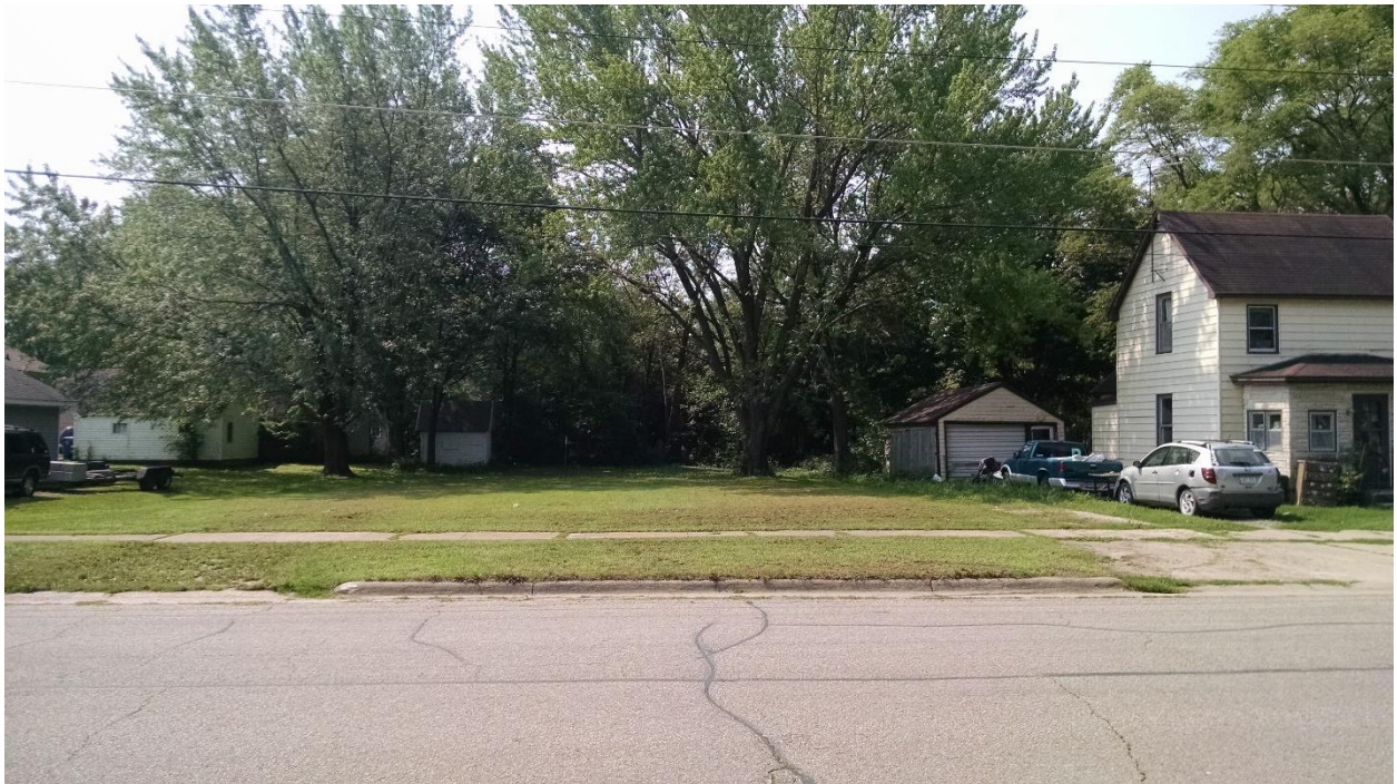
Cleared Site Following House Demolition – 312 15th Avenue
