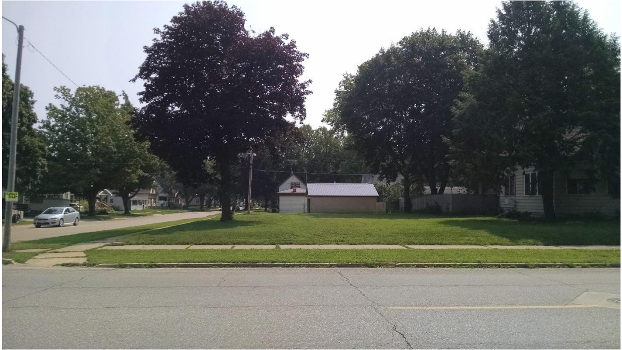
Cleared Site Following House Demolition – 806 North Grand Avenue
