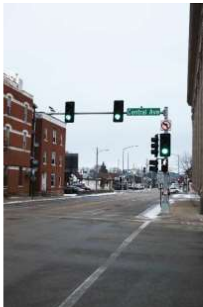
B. Non-Ornamental Municipal Service Pole
