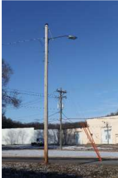
A. Existing utility poles
