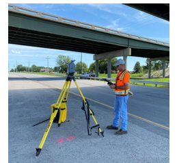
Surveying and Geospatial
