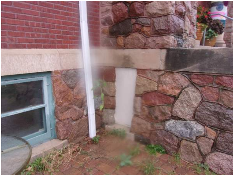
Figure 20: downspout discharge.
