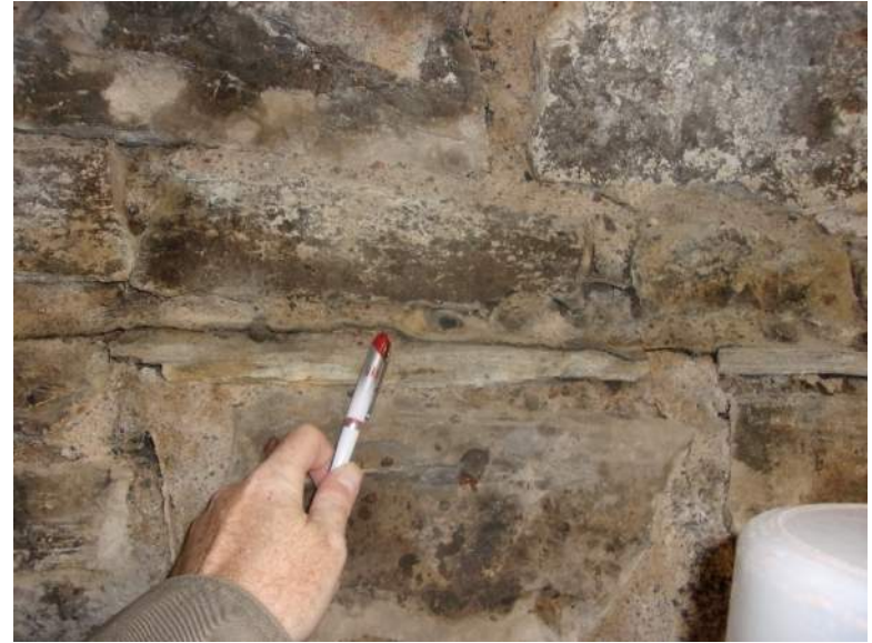
Figure 8: layer of flashing at exterior stone wall.
