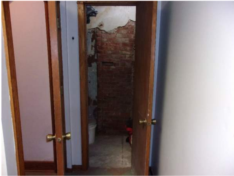
Figure 11: entrance to Men's toilet closet.
