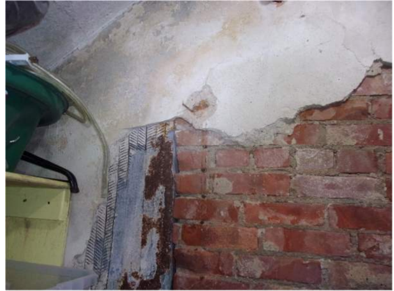
Figure 13: Men's toilet closet.
