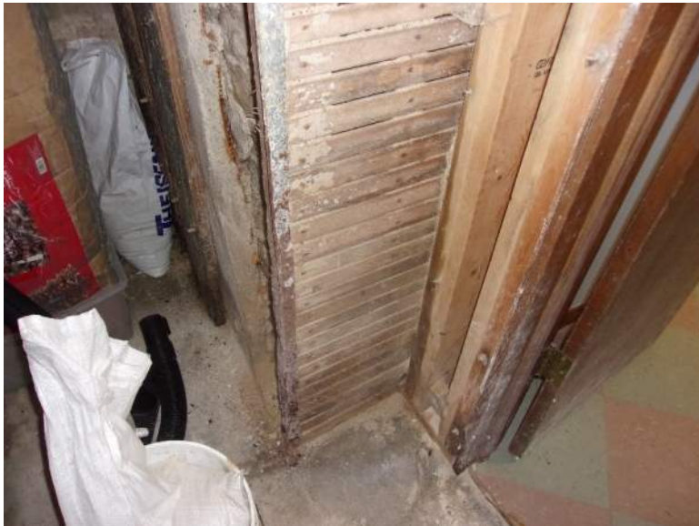
Figure 12: Men's toilet closet.
